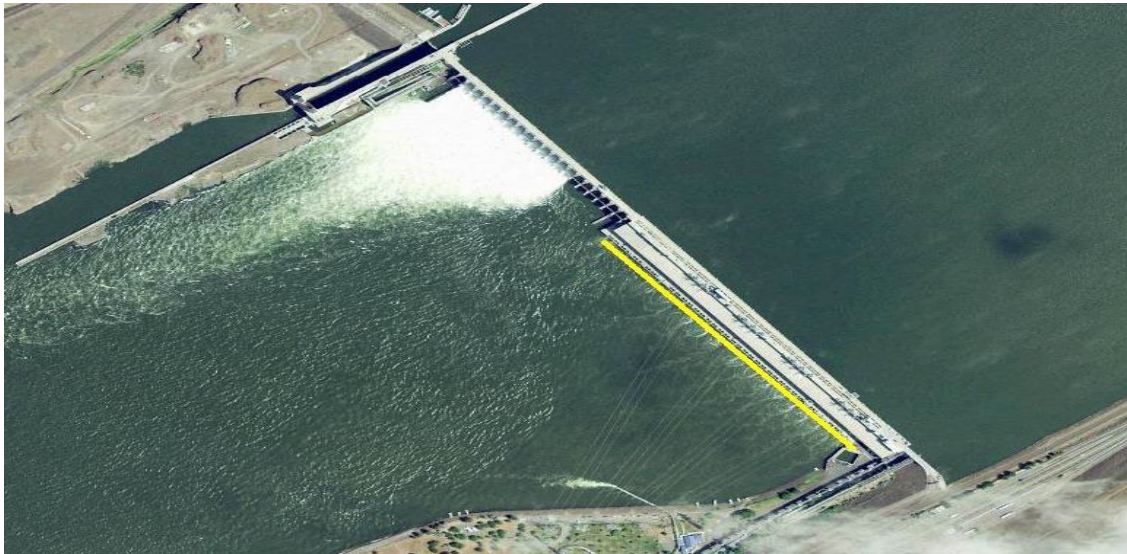
Figure 3. Angling locations for 2023 Dam Angling at the John Day Dam
