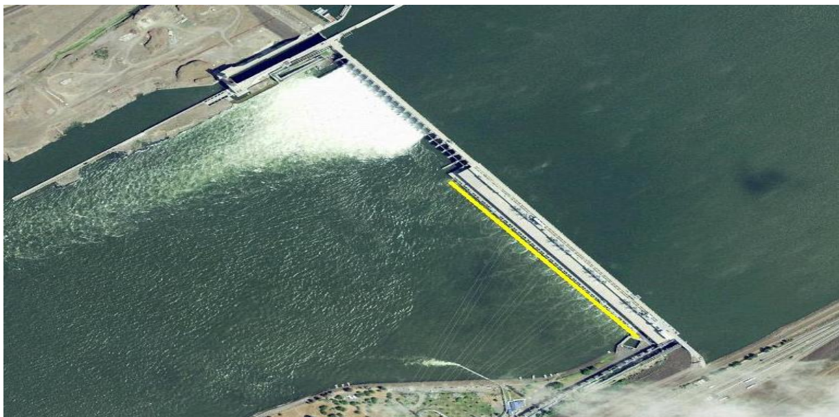
Figure 3. Angling Locations for the 2017 Dam Angling Crew at the John Day Dam
