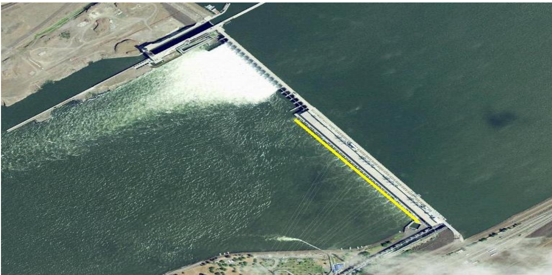
Figure 3. Angling locations for the 2013 Dam Angling crew at the John Day Dam.
