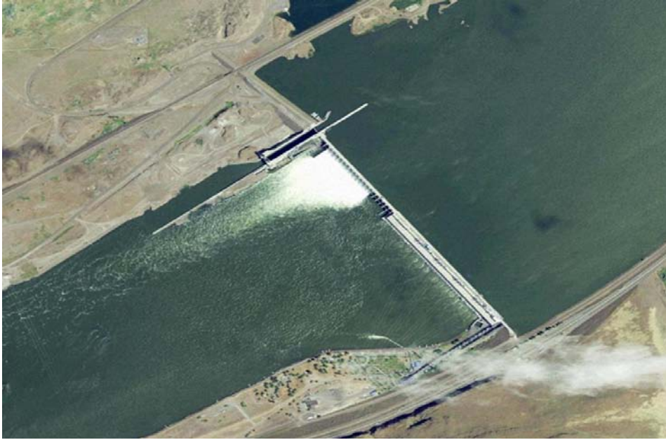
Figure 3. The John Day Dam.
